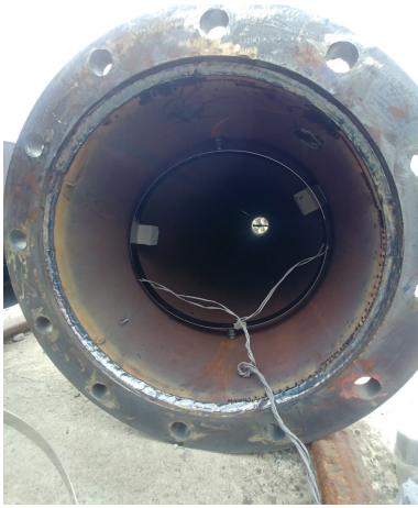
Fig. 13. Installation of circular displacement meter
