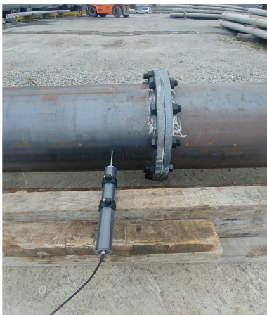
Fig. 14. Straight displacement meter installed externally
